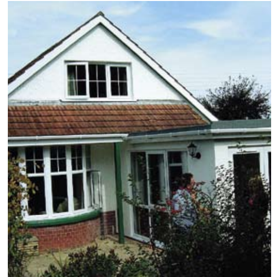
This attractive bungalow provides supported housing for three people in Barnstaple, Devon
